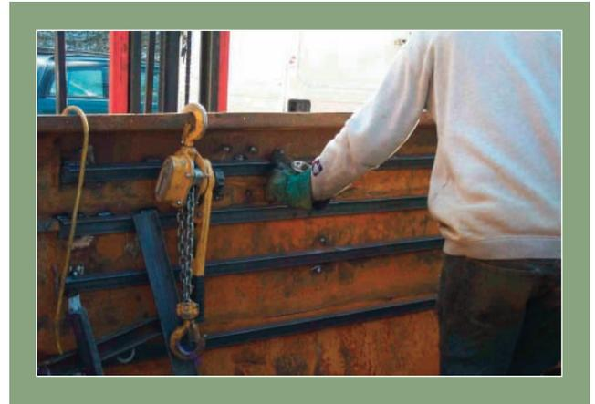
A moveable steel framework is then constructed. The framework holds a one and a half tonne winch or pulling block.
