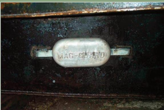
Four brand new anodes are attached below where the water line will be. A grinder is used to remove the paint, dirt etc. from the steel before the anodes are attached (providing a better contact).
