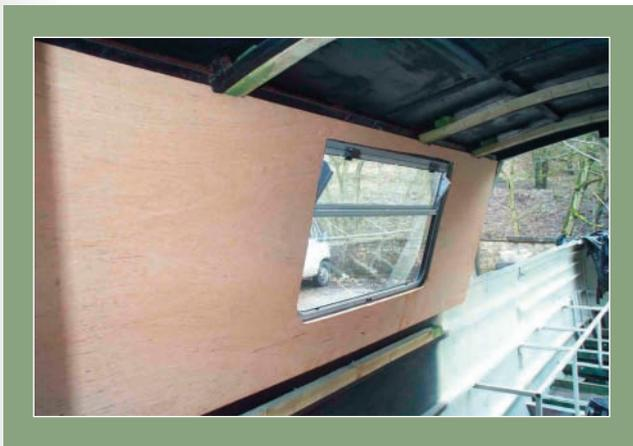
The plywood lining sheets are permanently screwed into place. The sheets have been attached to the vertical wall battens.
