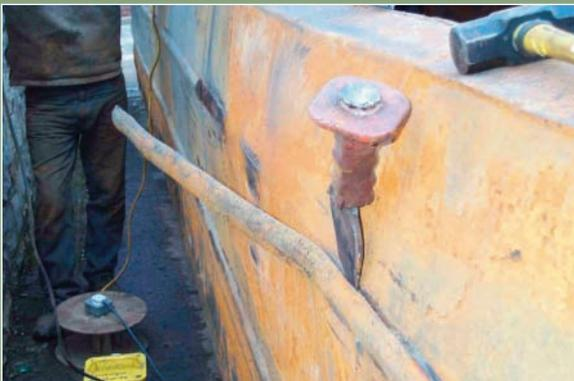
With a chisel, hammer and extra elbow grease the D-bar (rubbing strake) is painstakingly removed from the side of the boat.
