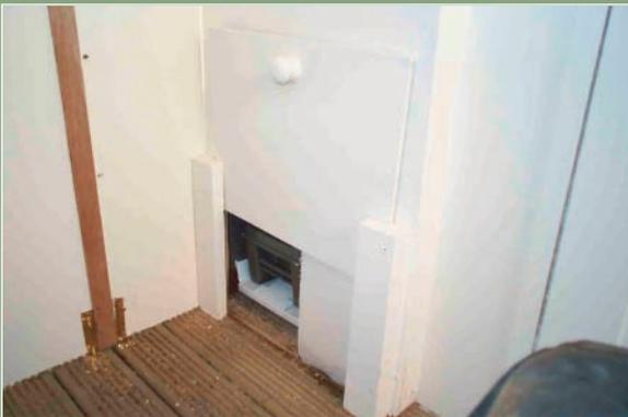
We start to board off the engine compartment. The stairs have been designed so that they can be removed if we need to get at the engine.
