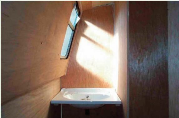
The sink is fixed into place against the back bulkhead. We realise later that the drain hole will be too low compared with the water line.
