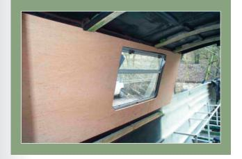
The plywood lining sheets are permanently screwed into place. The sheets have been attached to the vertical wall battens.
