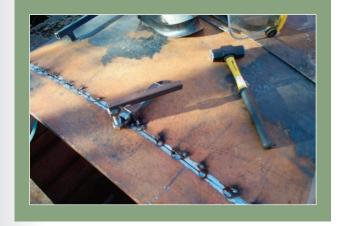
The two steel plates are pulled together and tac welded across roof and sides.
