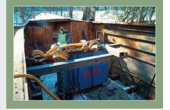
A moveable steel framework is then constructed. The framework holds a one and a half tonne winch or pulling block.
