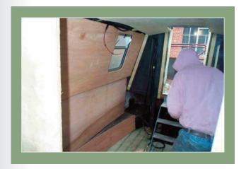
Work continues on the back cabin. The wire hanging from the ceiling is the power cable for the light in the toilet.
