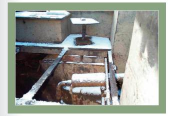
The diesel tank is drained off into five gallon containers. The diesel has a lot of water in it but this separates to the bottom of the container meaning you can filter the "good" stuff from the top.
